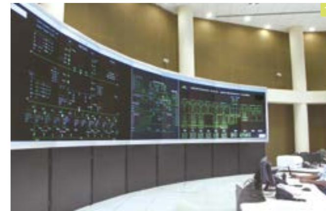
Bangalore Railway Traffic Control Center, India
